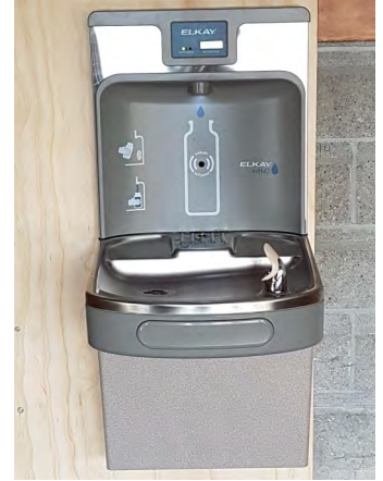
The newly installed water fountain in the dining hall
